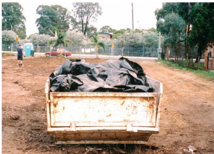
WRAPPED ASBESTOS WASTE
