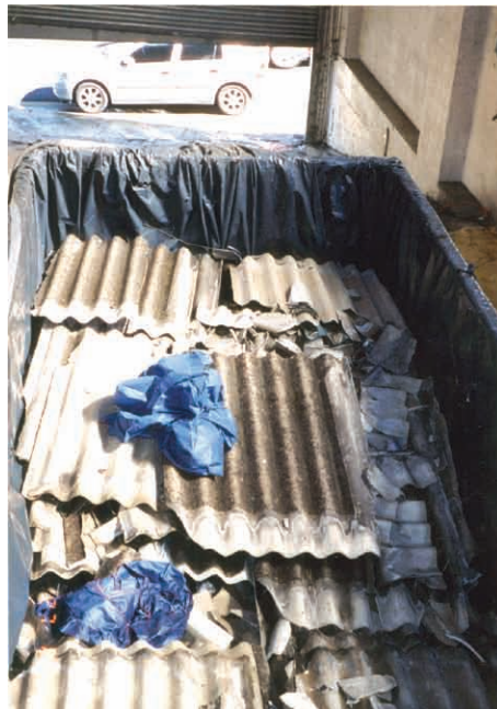
LINING BINS IN 200micron PLASTIC
